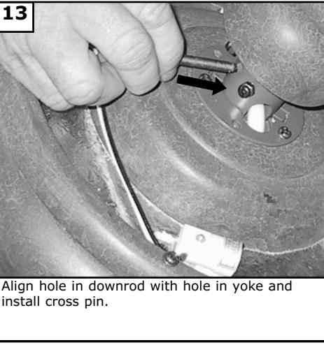
Align hole in downrod with hole in yoke and install cross pin.
